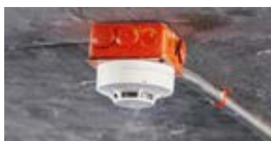
Other detection systems such as flame detectors and smoke detectors can also be used.
